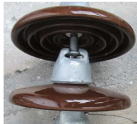
Gbr. 1 Isolator rantai 50 kV
