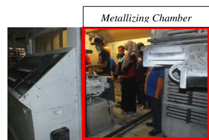
Gbr. 3 Metallizing chamber PT. Tomoko.
