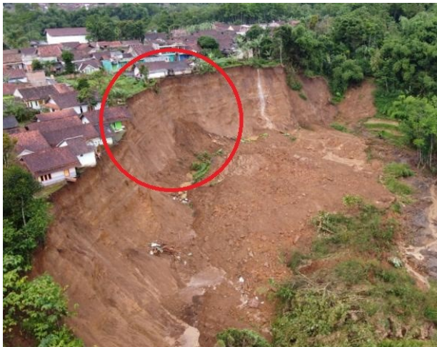
(a) Aerial photos
