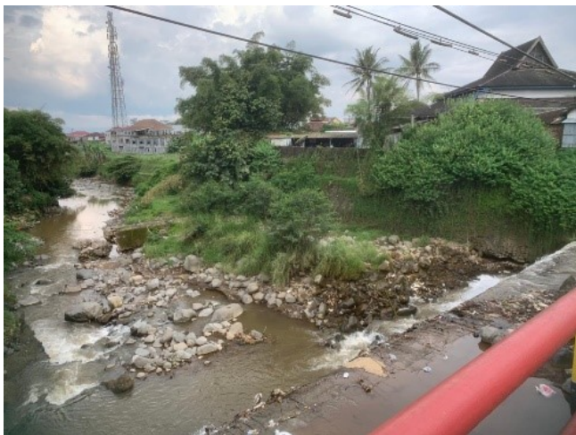
(a) Stream conditions at Galeh Bridge
