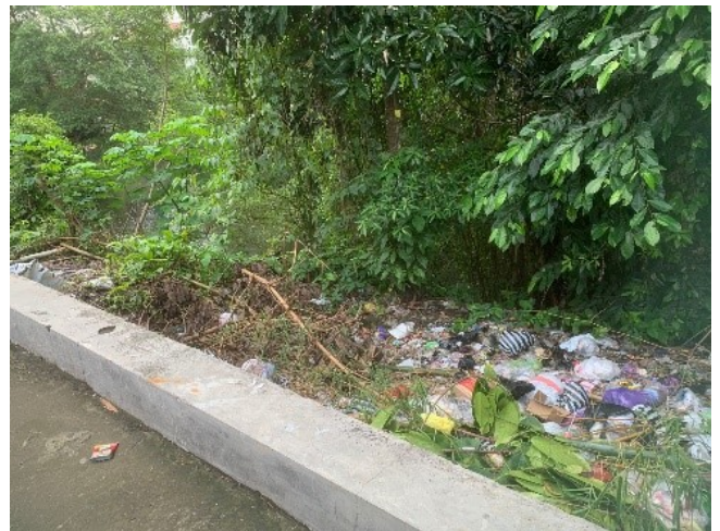
(b) Stream conditions at Gemping Bridge
