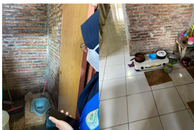
Figure 2. The bathroom and kitchen of one of the respondent houses
