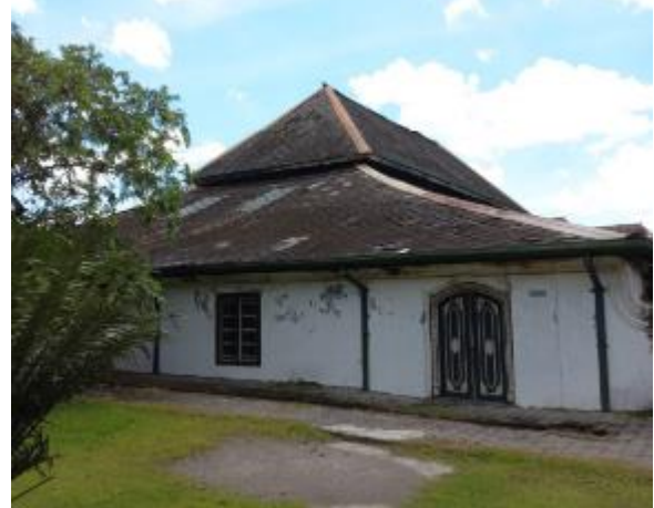
Figure 8. Front and Back View of Dalem Ageng Prabayeksa Source: Survey (2022)
