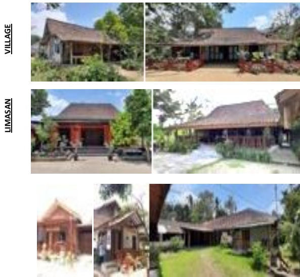
Figure 7. The majority of typologies of traditional building types are based on shape
