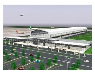
Another significant change from previously existed terminals is the use of glass as building's side wall. Usage of glass also made the efficiency on electricity spending by day because of natural sunlight that goes straight into the building so the usage of lamps can be reduced. There is also change saw on the colour palette usage, which is dominant turquoise for the walls and yellow for the signage, marking the modern era of simple and functional building.
