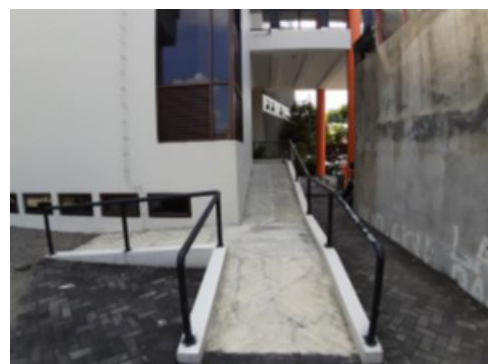
Figure 3. Ramp as a supporting facility for wheelchair users in the FISIP UAJY building
