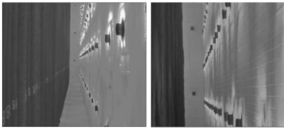
Figure 6. Radiant wall in hot condition before coating (left) and after coating (right).
