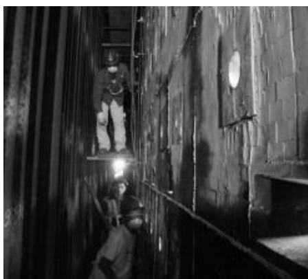
Figure 2. Scaffolding installation
