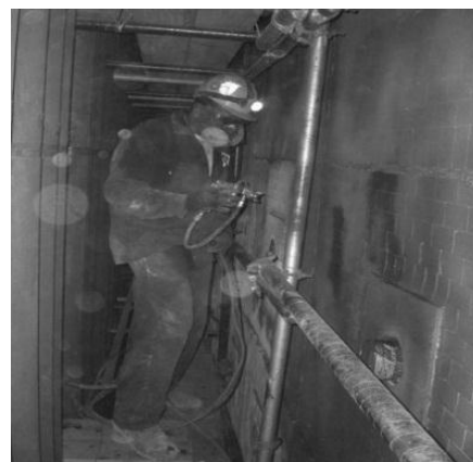
Figure 4. Application of coating
