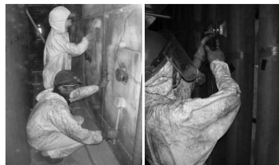
Figure 3. Brushing reformer tube and re-fractory surface hand brushing
