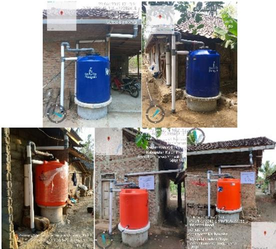
**Gambar 2. Alat GAMA Rainfilter**
