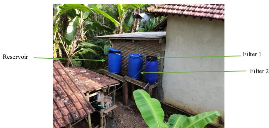
**Figure 3.** The results of the installation of the filtration system clean water treatment technology.
