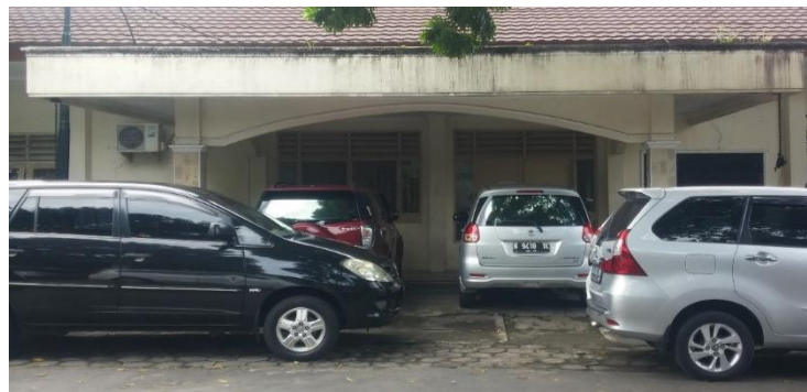
Figure 4.7 Access to entrance of PKSDA building blocked by vehicle
