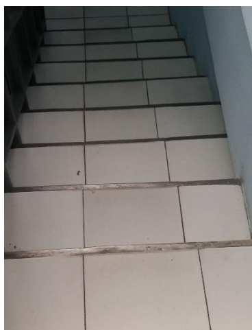
Figure 4.9 Stair in Water Resources Management Building
