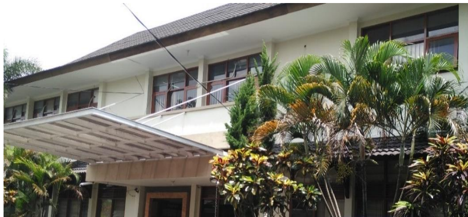
Figure 4.1 Side of the Serayu Opak River Basin Organization building
