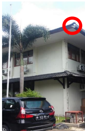
Figure 4.2 Rainwater gutters without vertical pipes at Serayu Opak River Basin Organization building
