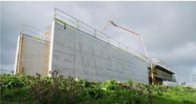
Figure 10. Full scale demonstrator in situ cast self-healing concrete water reservoir (Mors & Jonkers, 2019).
