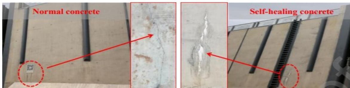
Figure 13. Comparison of self-healing effects of ship lock wall made by normal concrete (left) and made by bacterial concrete (right) (Zhang and Qian, 2020).
