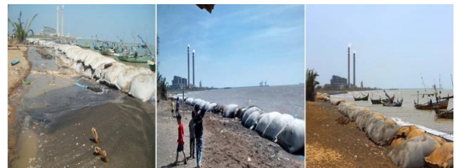
Figure 13. Construction of low-crest breakwater in Jepara Regency
