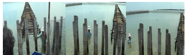
(b) Geobag Low-crest Breakwater with Bamboo Poles
