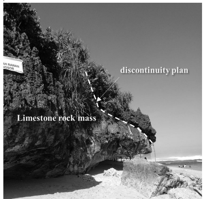
Figure 3. Potential slope failure in Sadranan Beach
