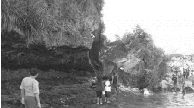
Figure 1. The rockfall incident on 17th of June, 2015 (Kusuma, 2015)
