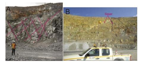
Figure 4: Joints and faults observed in research area.
