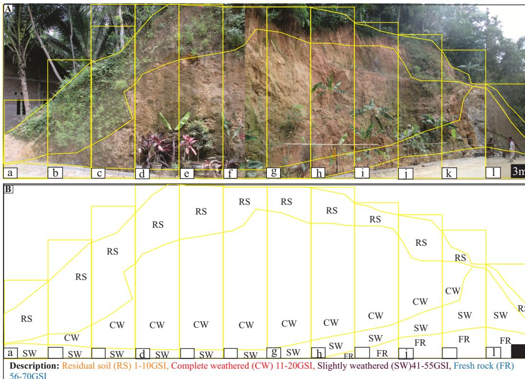
FIGURE 3. Overall view of the Kalirejo Road Side Slope: (A) Photograph of the slope; (B) Weathering profiles.
