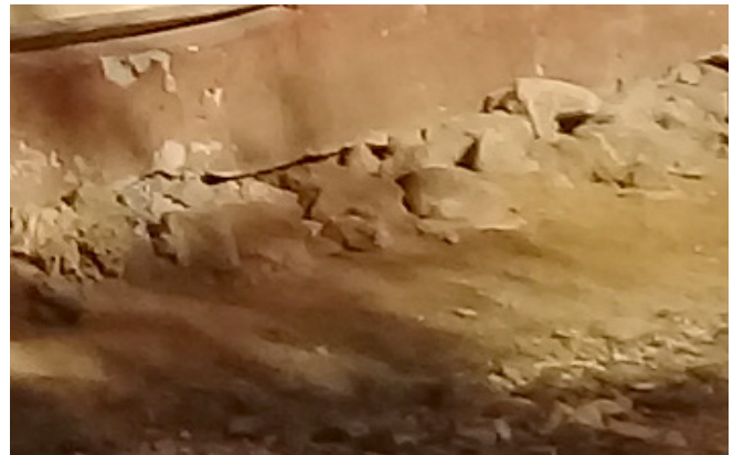
Figure 10. Exposed tree roots and eroded building foundations structure in land unit L0b5A with density-housing land use. Soil loss by field indicators was 57.97tons/ha/yr, and by RUSLE was 110.72tons/ha/yr. Land degradation rate by erosion was categorized high
