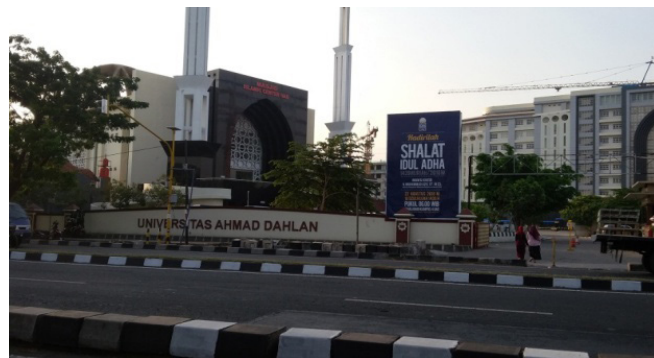
Figure 3. The Ongoing Construction of the Ahmad Dahlan University Campus in Tamanan Village
