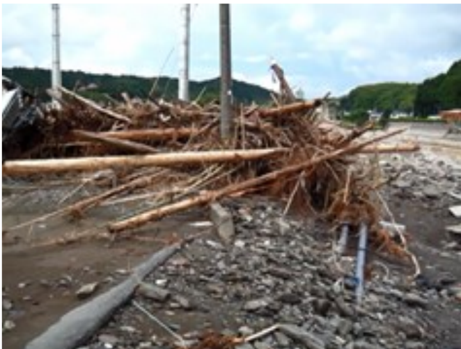
Figure 16. A woody debris jam at utility poles at ‘Yamauchi’ district and A woody debris jam at three different trees at ‘Funagoya’ district
