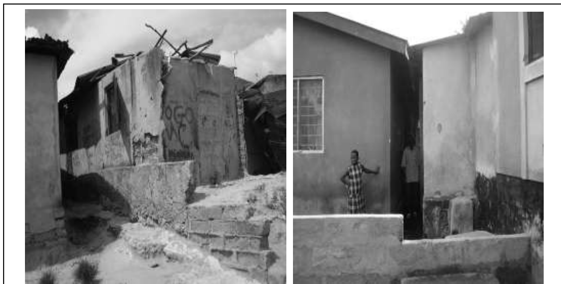
Figure 5. Houses very close to each other with very limited access
