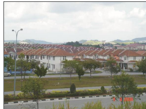
Figure 9. A typical double storey terrace housing in Malaysia
