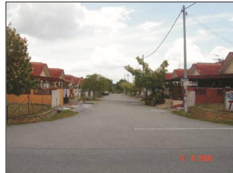
Figure 8. A typical single storey terrace housing in Malaysia
