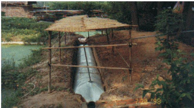
Figure 1. A low-cost digester made of polyester tube in Vietnam as an option (Bui Xuan An and Preston, 1995)
